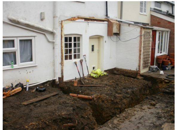
DP10: Post-excavation of the foundation trenches, facing NE.
