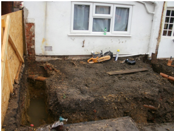
DP9: Post-excavation of the foundation trenches, facing NW.
