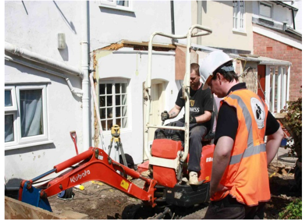
DP8: Archaeologist monitoring excavation of foundation trench.
