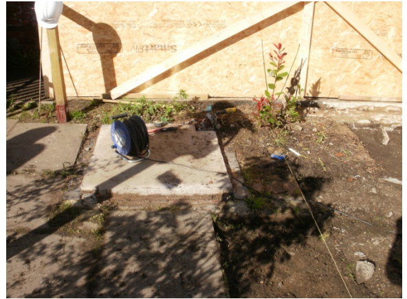
DP4: Shot of Victorian toilet block and brick work, facing NW.
