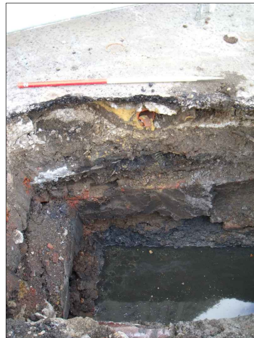
DP5 - TEST PIT 3 SAMPLE SECTION VIEW NE
