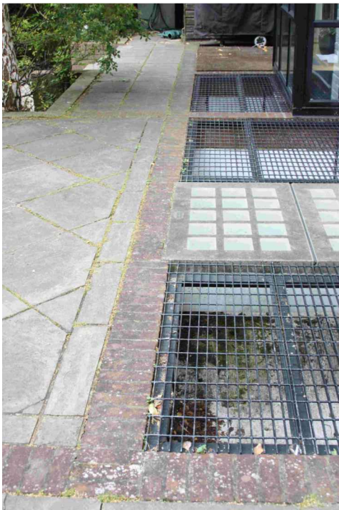
Photo 4: Light wells for Existing basement
